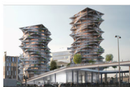
Kaktus Towers, Copenhagen SEK 1 334 M *
